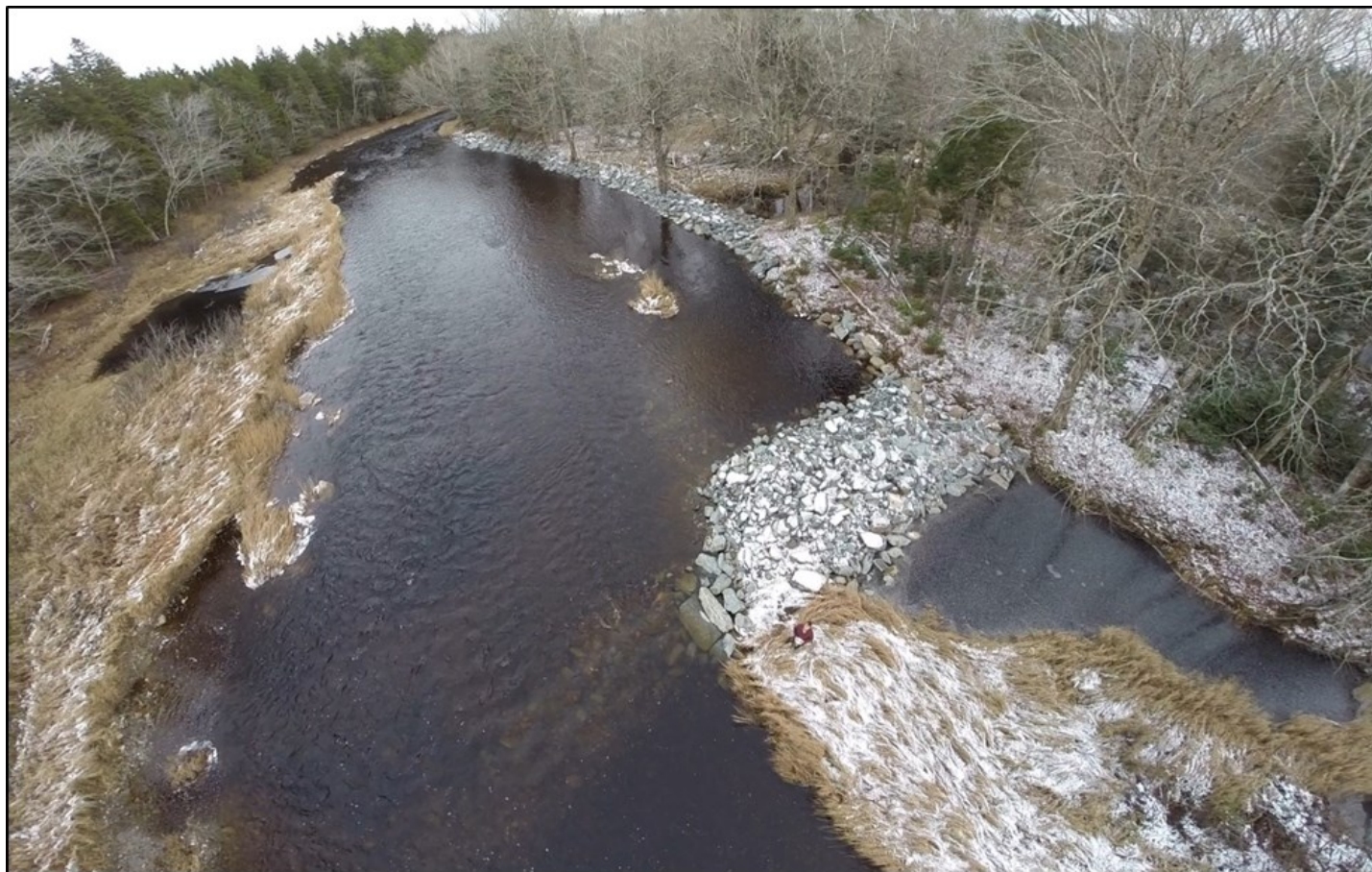
West Branch view of restoration work, bank protection, channel blocker and sill. Photo credit: Nicholas MacInnis.
