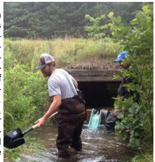
Fish passage NSLC Adopt A Stream field technician, Will Daniels worked with UINR to fix fish passage on Bryden Brook CB. Wooden baffles and a fiberglass chute were installed in a box culvert.
