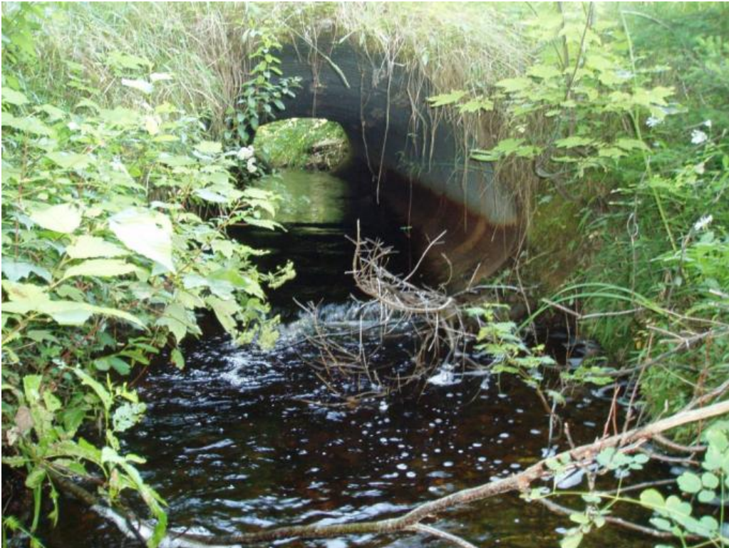
Plate 5: Inlet of paired arch pipe culverts (upper) and outflow of one of these culverts (lower) on Hattie Brook (Culvert #68).
