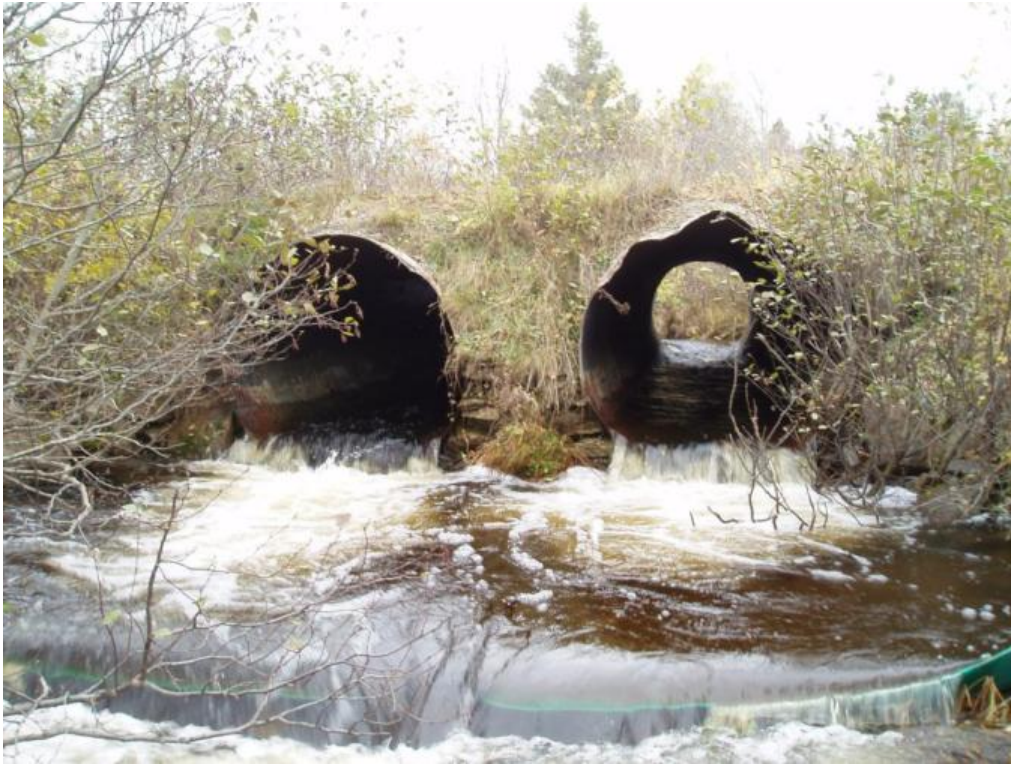
Plate 2 (cont'd): Culvert on Fraser's Brook (Culvert #96) at high flow; Note green plastic weir submerged in flow.
