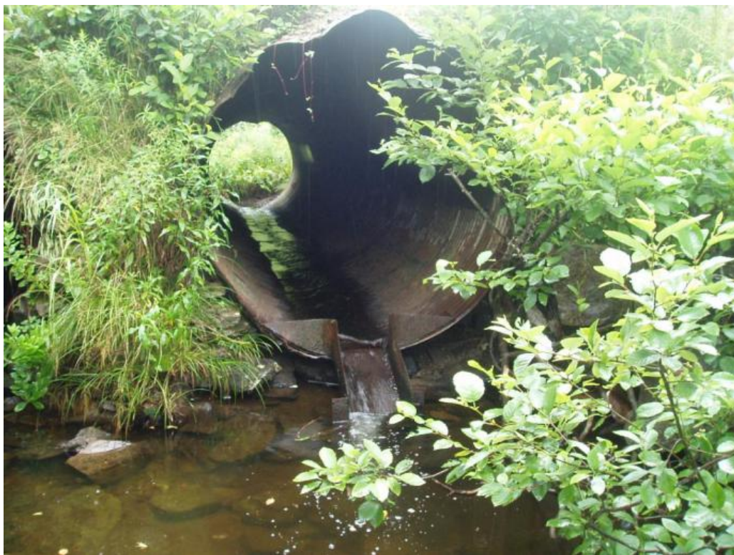
Plate 2: Outflow culvert on Fraser's brook (Culvert #96) at low flow; showing spillway intended for fish passage.
