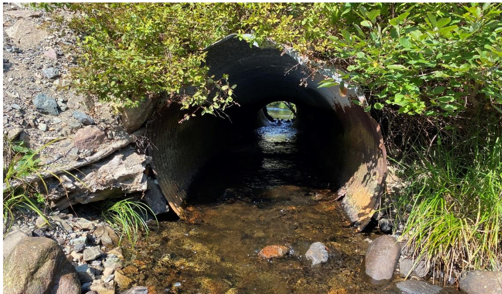
Figure 12: Looking upstream through the main culvert. Partial fish passage was available at this time (Sept 2021).
