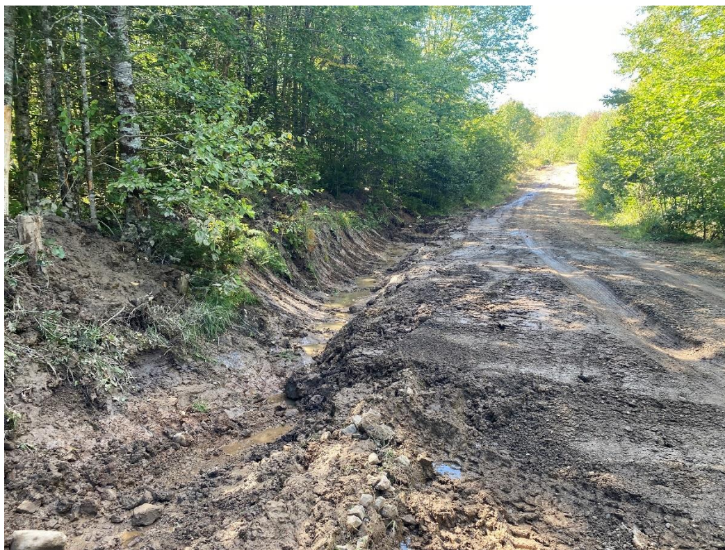
Figure 29: Forestry Road construction creating siltation near the Greens Brook - Black Brook confluence.
